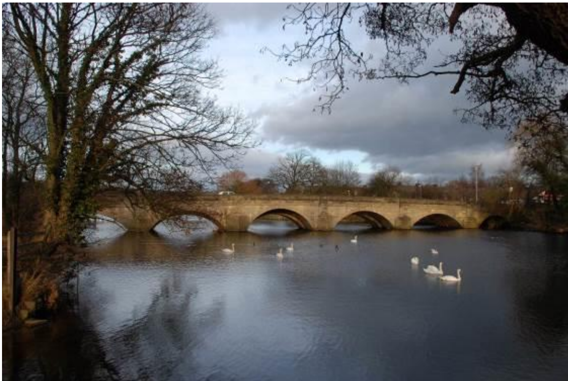
Bridge over the River Wharfe at Otley
