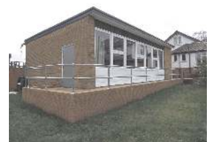
The new wheelchair ramp at Roundhay Meeting House
