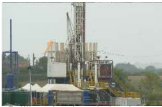
Drilling rig already in place at Kirby Misperton
