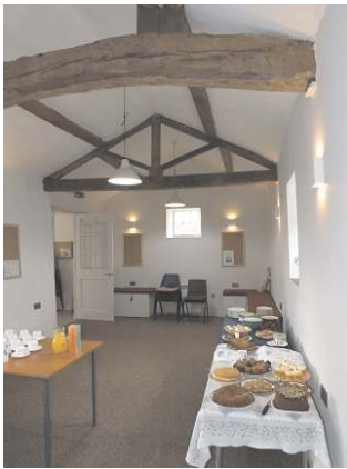
The School Room, with the newly refurbished roof beams.
